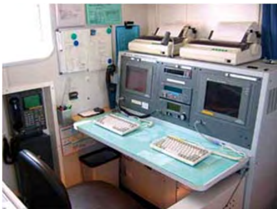
無線区画－1／Radio equipment area-1
